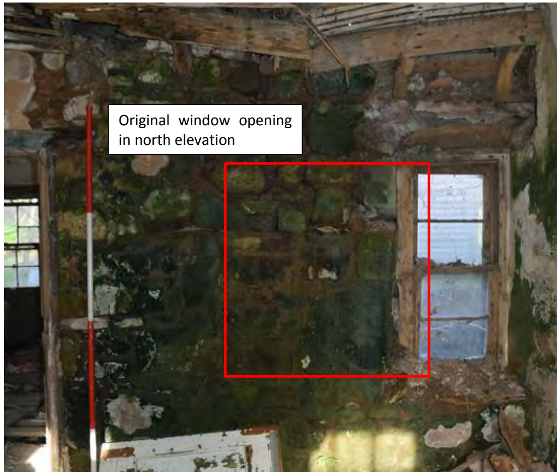
Plate 18: Blocked and inserted window in north wall of the original structure (Cottage 1, Room 4).
