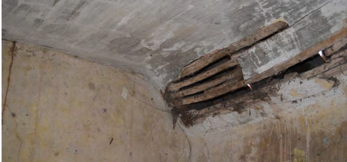
Plate 21: Lath and plaster coved ceiling.
