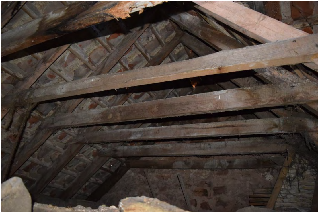
Plate 22: Main A-frame roof timbers with carpenters marks in the original cottage.
