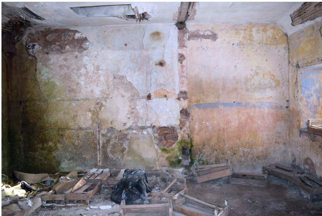
Plate 17: Walls plastered on the hard and showing scars of brick partition walls (Cottage 1)
