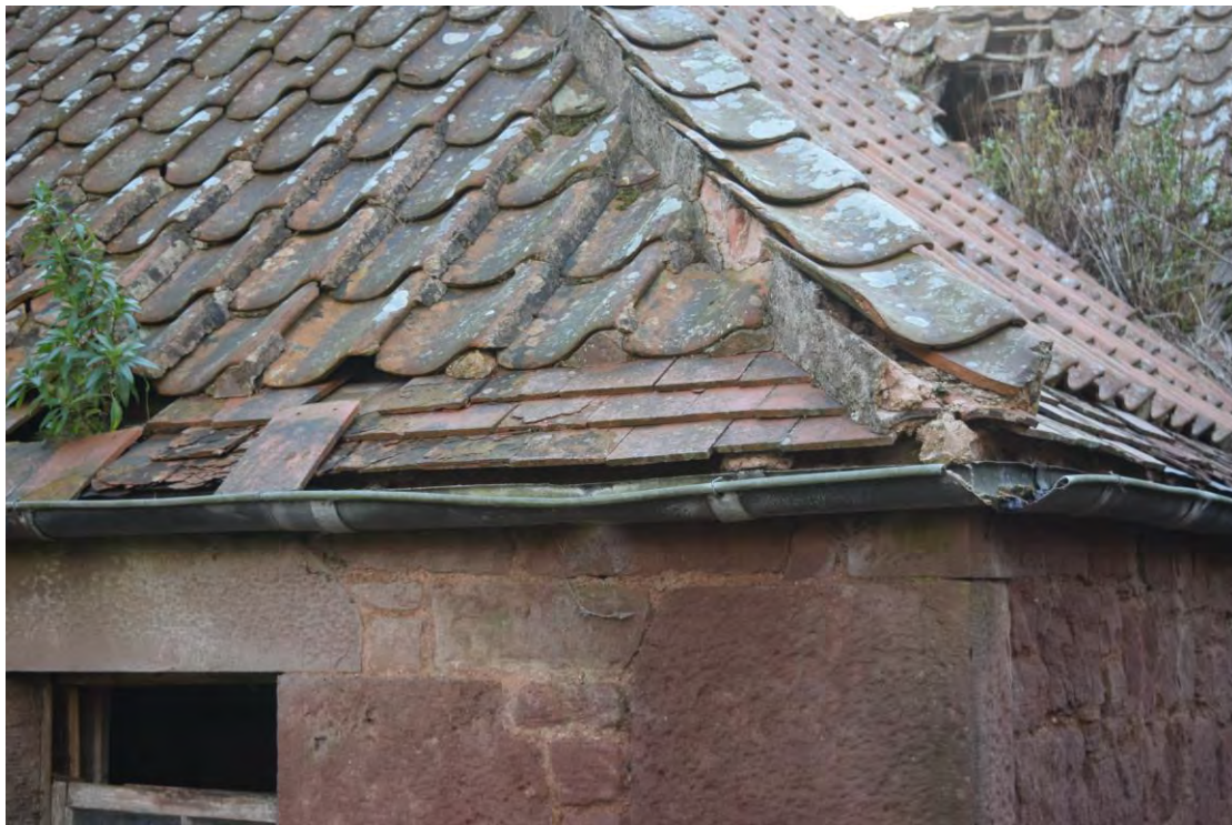
Plate 16: Roofing on cottages (north elevation), with clay tile easing courses and pantile ridge.
