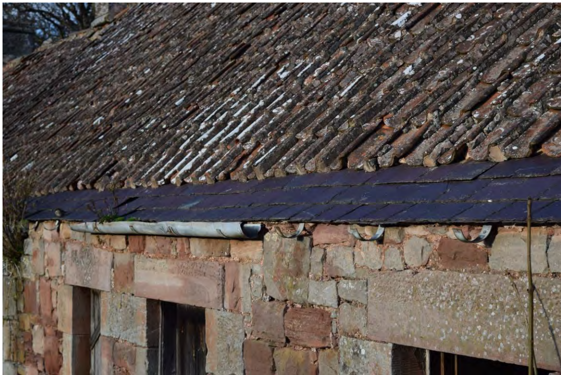
Plate 15: – Roofing on cottages (south elevation), with slate easing courses
