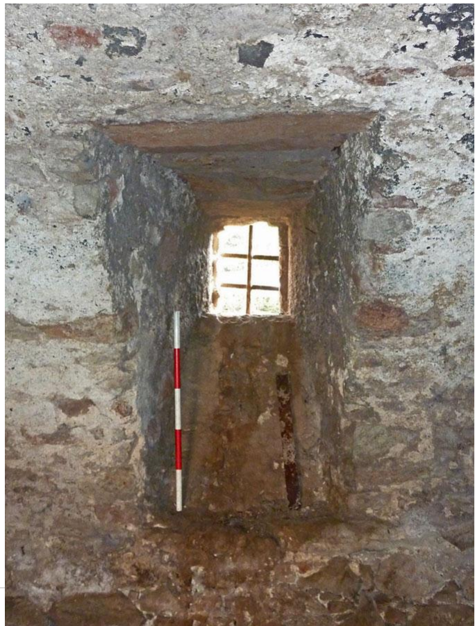
Plate 6: Original window with bars in vaulted Room 4
