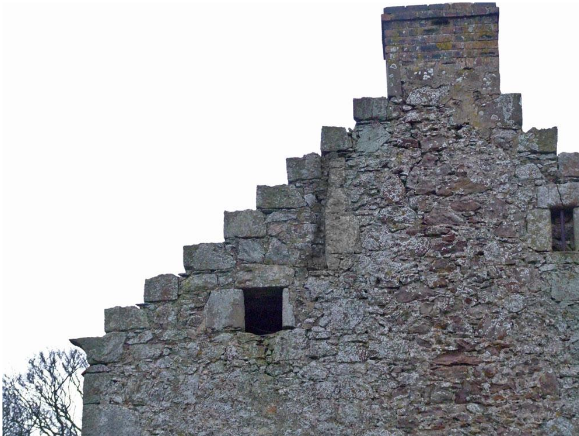
Plate 2: East gable elevation with truncated earleir window beneath crowsteps
