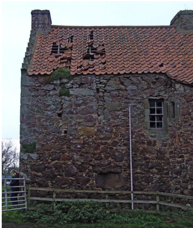
Plate 3: west end of south elevation showing complex sequence of window openings, insertions and blockings
