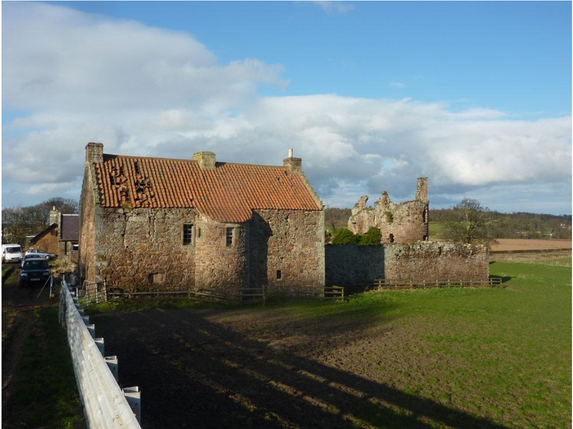
Plate 19: View of the southwest lodge and castle from the south
