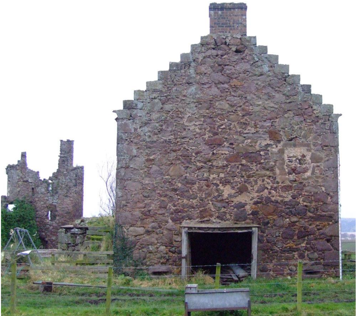
Plate 4: West gable with large central ground floor opening and original window on 1st floor to the right - now blocked. The castle ruin is in the background.
