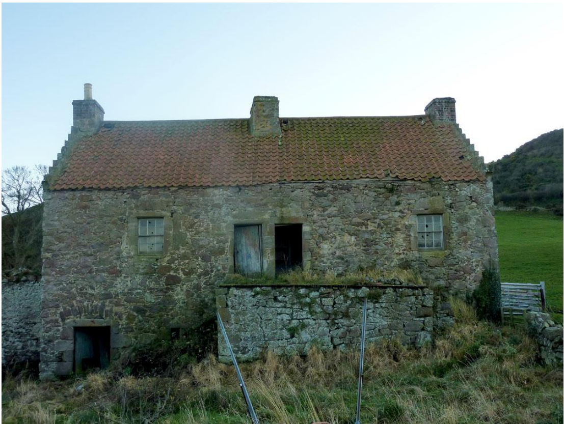
Plate 20: The north elevation with platform providing entrance to the workers cottages
