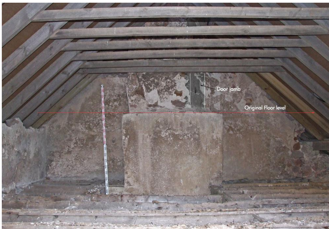
Plate 7: Room 18 roofspace with original floor level for the second floor marked and the original doorjamb highlighted.
