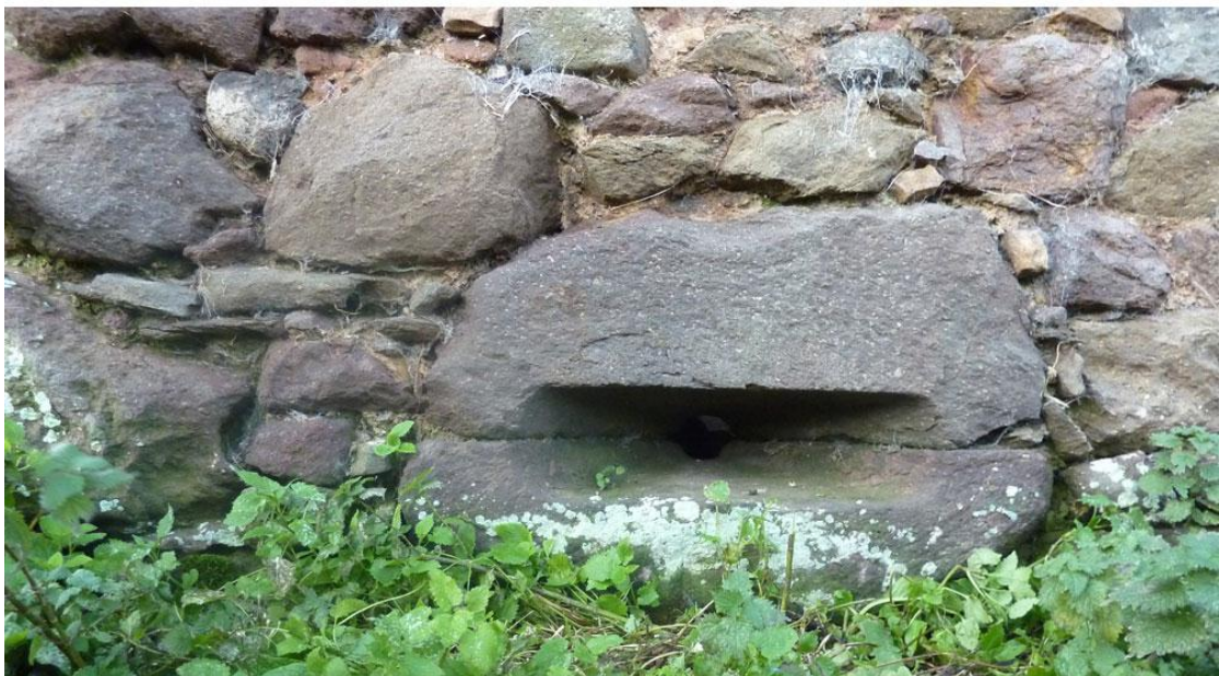
Plate 10: Internal and external view of gunloop.
